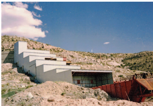
Figure 1. Western General Resources mill constructed late 1970's at the Blanchard mine. DeMark photo, 1987.
